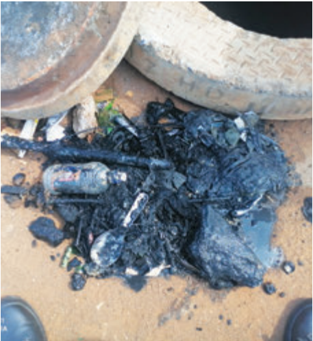
TLM spend two days inside the drains to unblock the sewer system.
